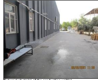
External photo(s) of the production unit(s) fire hose tested.jpg
